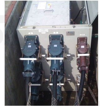
Cruise vessel connection box at shore
