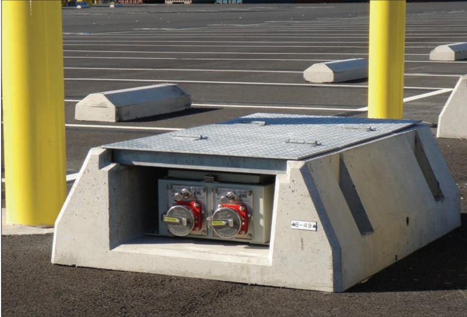
outlets per bunker, or possibly on upright pedestals which provide easier access to the receptacles but are also more susceptible to damage by trucks and other yard vehicles. Pedestal designs sometimes incorporate protective bollard systems; these are expensive
