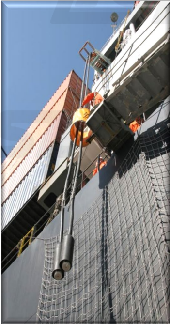
Cable management system on board container vessel
