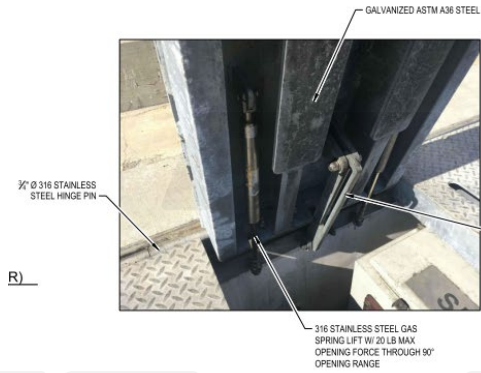
1 VAULT LID FEATURES (OPEN) SCALE: NTS
