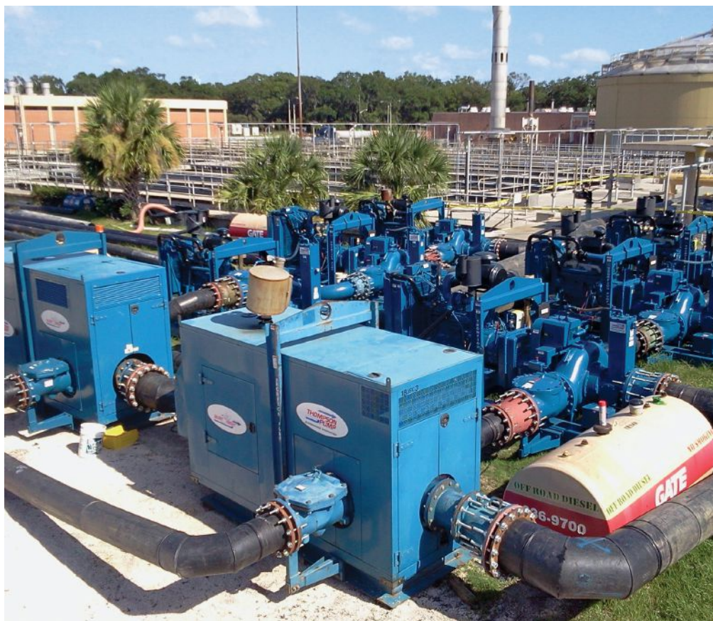
A sewer bypass at the Buckman Waste Water Treatment Plant in Jacksonville, FL
