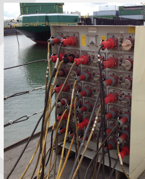
20-Gang Modular RSU Assembly ESL Series: 3500-02
