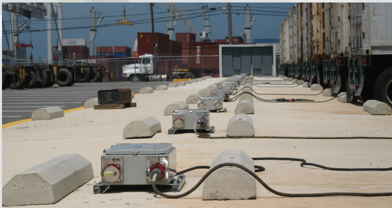
4-Gang Bunker Mount Assembly ESL Series: 2207-88
