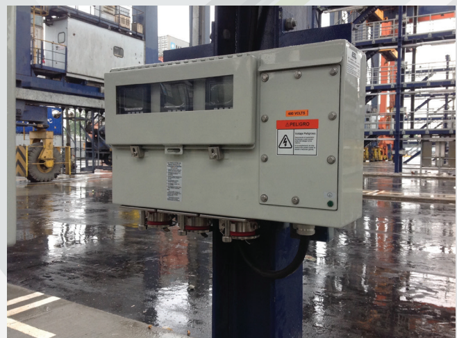
3-Gang Rack Mount with Energy Meters ESL Series: 2223-07N
