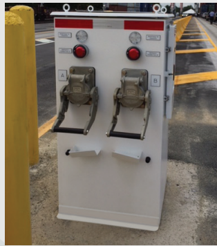
ERTG Disconnect Cabinet 1000V 700A 50/60Hz ESL Series: 5101-36E
