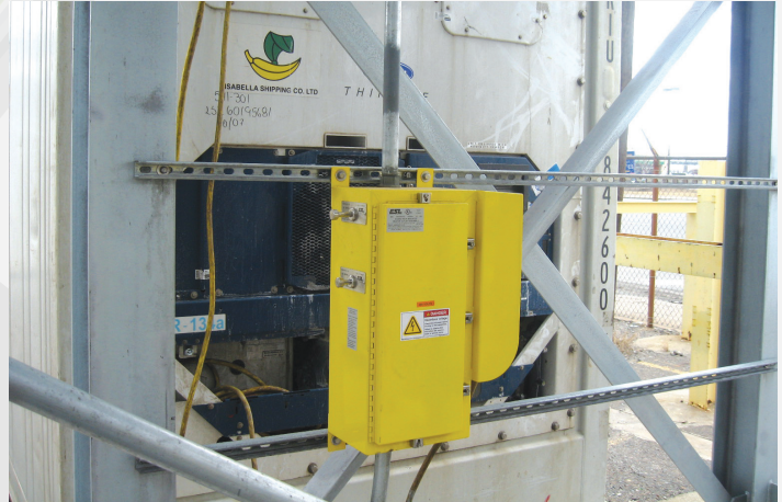
2-Gang Rack Mount Rear Actuated Assembly ESL Series: 2221-14L
