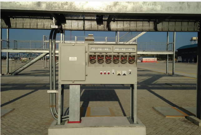
6-Gang Pedestal Mount Reefer Outlet Assembly ESL Series: 2222-77
