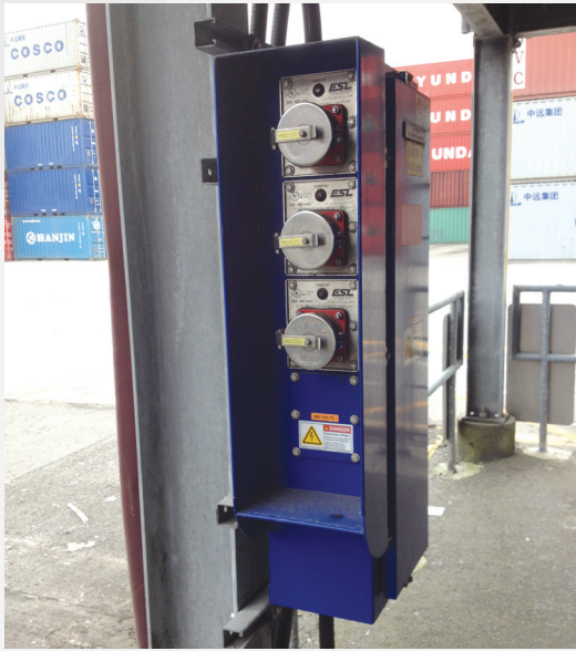
3-Gang Rack Mount Rear Actuated Assembly ESL Series: 2221-39L4
